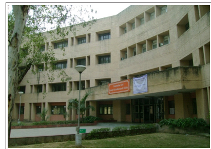
Construction Yard, Faculty of Architecture
